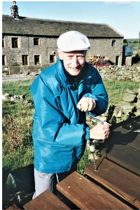
Jack at work, repairing a bridge at Bankfoot Farm, Timble 1996
